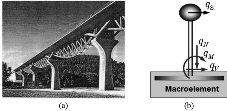
Fig. 5. (a) The columns of the Arc Viaduct in France (Design by Greisch Consultants) and (b) Simple model for dynamic analysis
