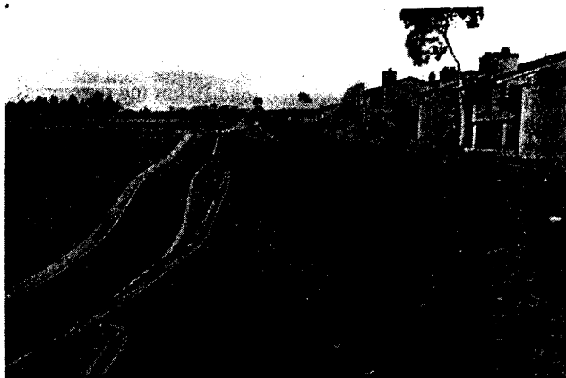
FIG. 13. Completion of Slope Shown In Fig. 12, with Erosion Control Fabric on Slope Face
